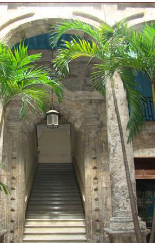
Stairs of the Palacio del Segundo Cabo ©Office of the Historian of the City of Havana (OHCH)
